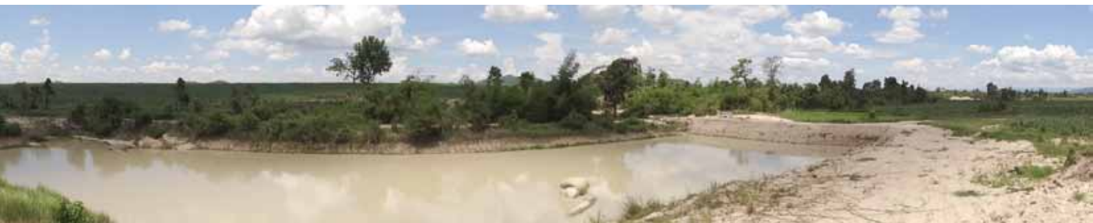
Picture 7: Company dam in concession blocks river to La'ngim Village
